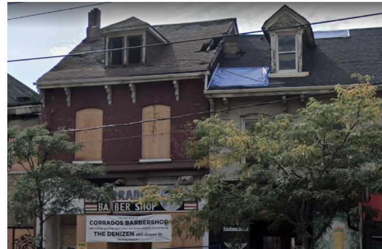
2014 - View of 160 to 164 Bathurst Street, showing the configuration of storefronts at grade, paired brackets with simple cornice, dormers, and high gable roof pitch of 162 and 164 Bathurst. Fire damage to 160 Bathurst Street resulted in removal of the property, and damage to a portion of the building at 164 Bathurst Street (Google)
