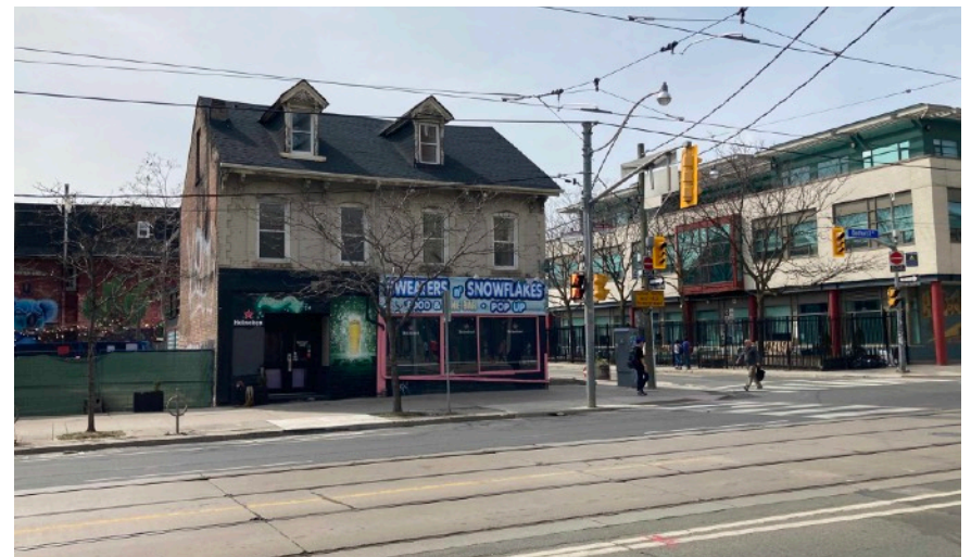
View of the subject site looking west along Bathurst Street towards the intersection at Richmond Street. To the north is the three-storey Central Toronto Community Health Services building. To the south side is 164-166 Bathurst Street which has been evaluated as having cultural heritage value and will be integrated into the proposed development. Fire damage from a 2019 fire is visible on the south elevation.
