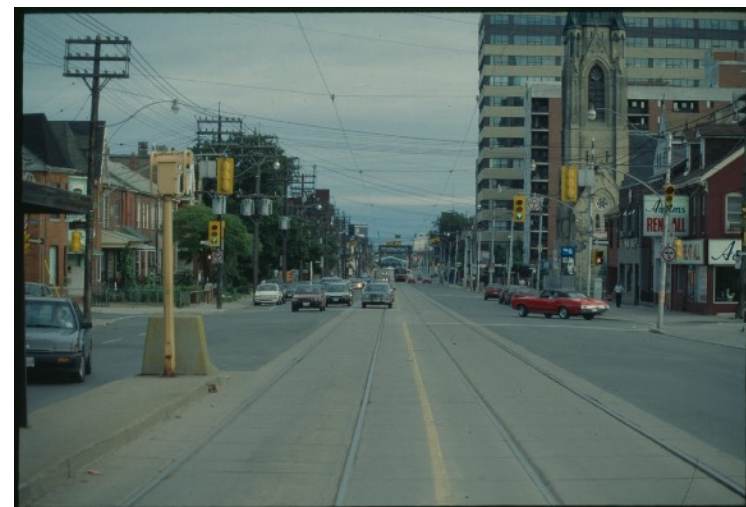
City of Toronto Archives, Series 1465, File 514, Item 6 1983 to 1985 - View of Bathurst Street looking south from Public Lane north of Richmond Street. The subject site can be seen on the right side of photograph, 164 Bathurst Street occupied by 'Adam's Rent-All' commercial storefront.
